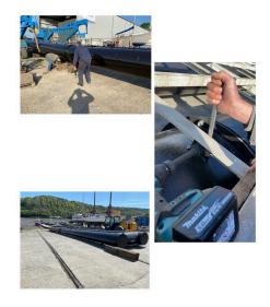
9. The two hammerhead floats were joined together using new high tensile bolts.
