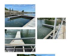
5. All pontoons were reconnected using new 100mm x 50mm rubber joining blocks with stainless bolts and nyloc nuts with large heavy duty washers.
