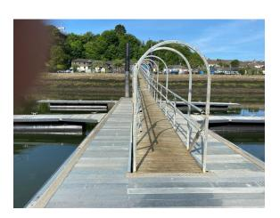
7. Final fitting of deck boards relayed and 6mm aluminium checker plate fitted across access pontoon to Hammerhead pontoon.
