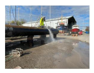
3. "hydro-blasting" was used to removed all protective coatings back to bare metal.
