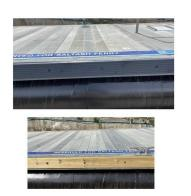
10. New Tantalised wood Pontoon fenders fitted to all sides of pontoons and coated in grey with new stainless nuts & bolts.
