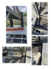
6. On the lift of tide and use of chain blocks the RSJ iron grinder was removed with Safty chains from under the access bridge and lowed onto the access pontoon
